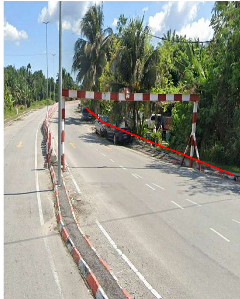
JALAN MISDI (OPEN CUT)
