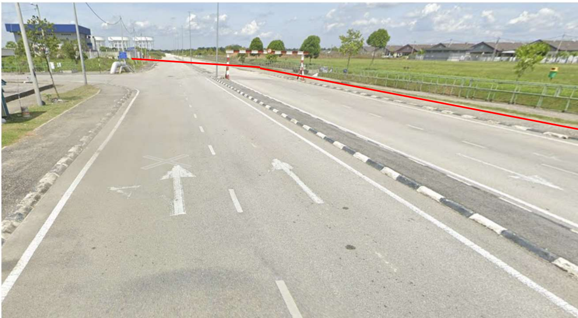
JALAN MISDI PPU TAMAN LAGENDA (OPEN CUT)
