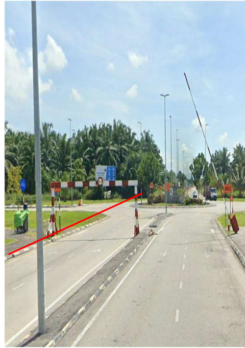
JALAN MISDI (OPEN CUT)
