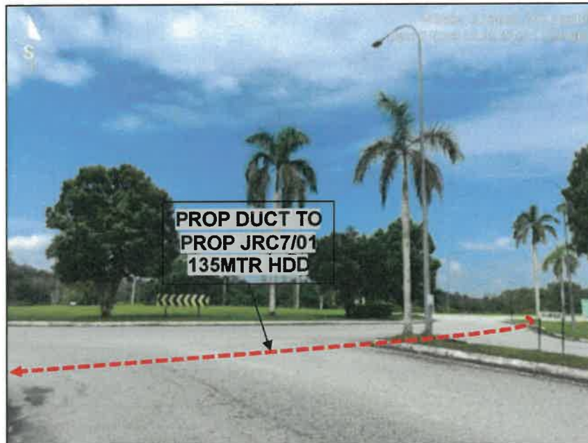
PICTURE 04: LOCATION AT JALAN PC10
