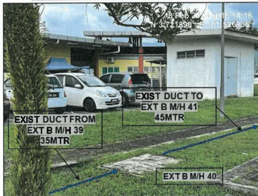
PICTURE 50: LOCATION AT UNNAMED ROAD
