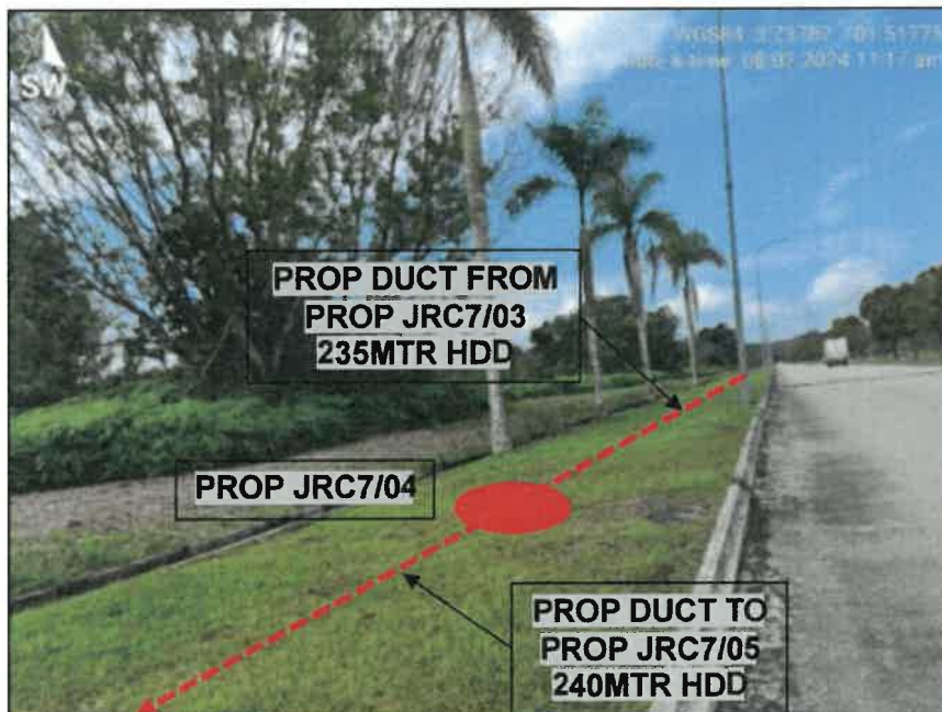
PICTURE 08: LOCATION AT JALAN PC10
