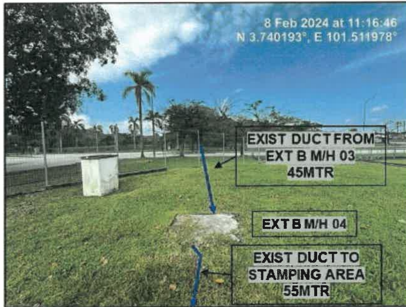
PICTURE 05: LOCATION AT STAMPING AREA BUILDING
