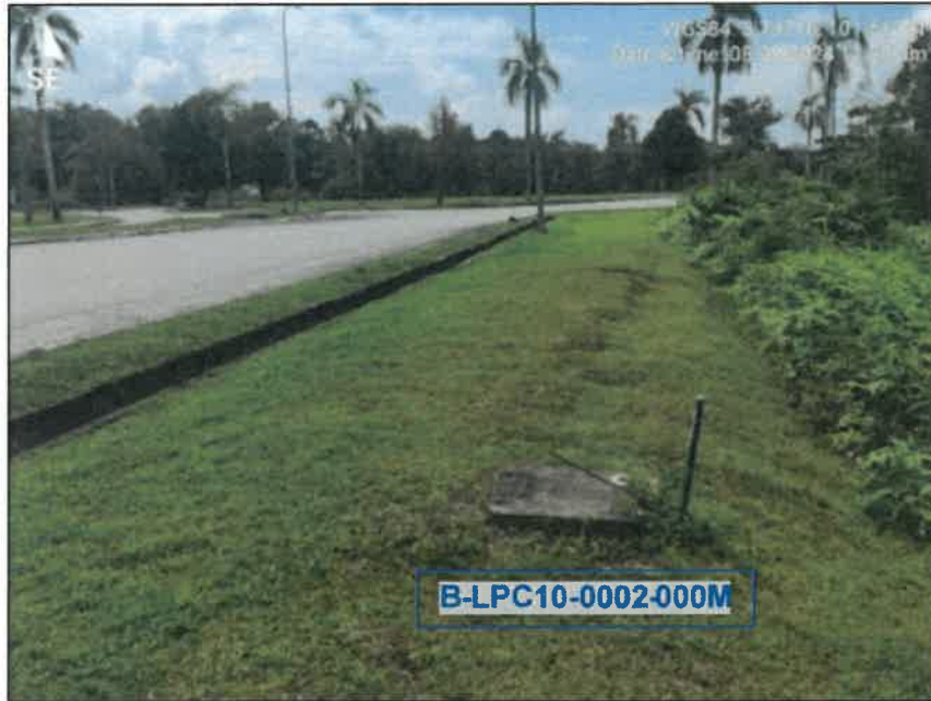
PICTURE 01: LOCATION AT JALAN PC10
