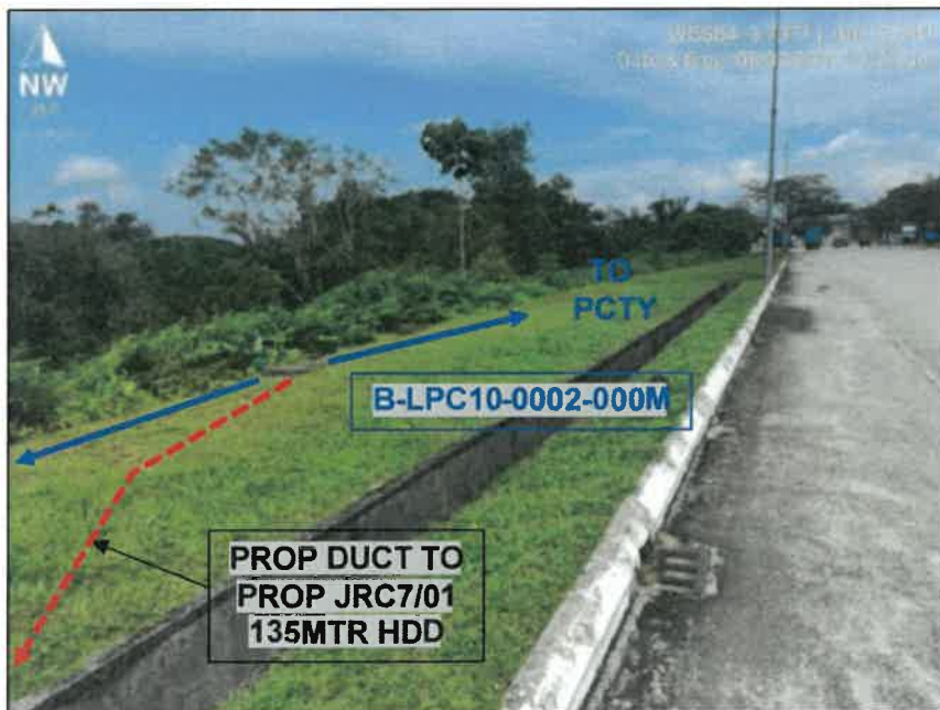
PICTURE 02: LOCATION AT JALAN PC10
