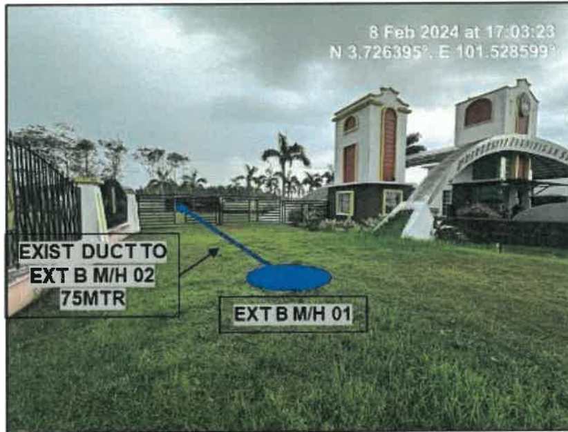
PICTURE 11: LOCATION AT ENTRANCE UPSI
