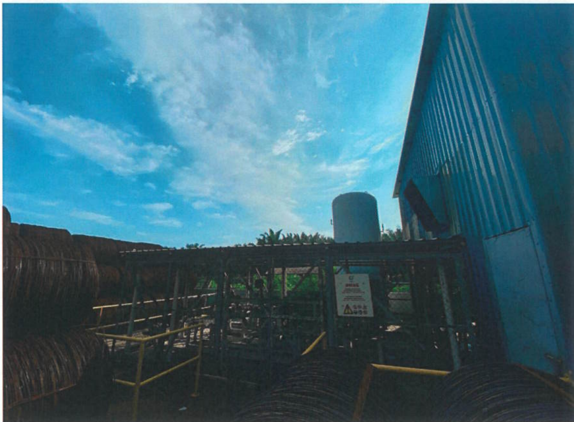
Figure 2: Existing station F500 to be demolished
