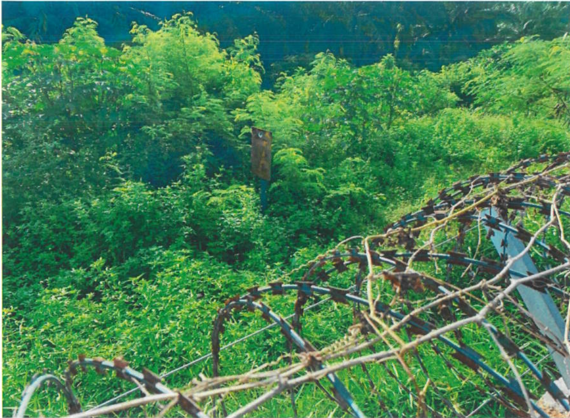
Figure 1: Proposed take-off point for the proposed pipeline (NPS 4) using hot tap from existing service line (NPS 4)
