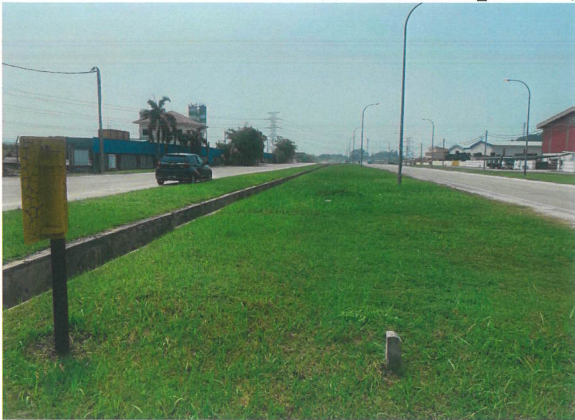
Figure 1: Proposed take-off point for the proposed pipeline (PE 125mm) from existing end cap (PE 125mm)
