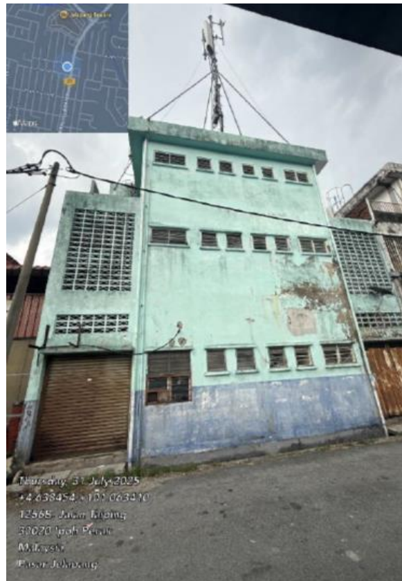
PICTURE 8 : EXISTING MH BUILDING
