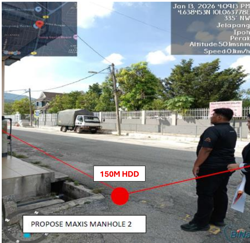
PICTURE 6 : PROPOSE 250M HDD TO PROP MH02
