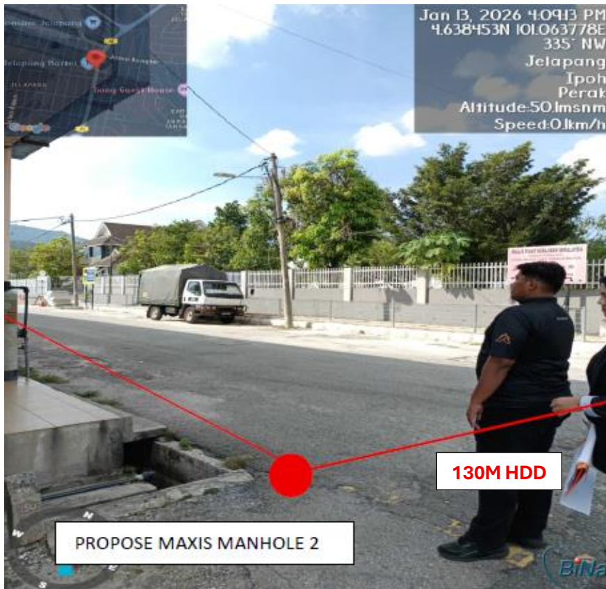
PICTURE 6 : PROPOSE 130M HDD TO PROP MH02
