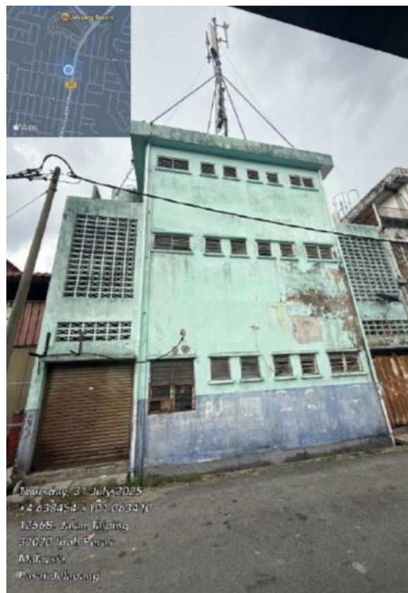
PICTURE 8 : EXISTING MH BUILDING
