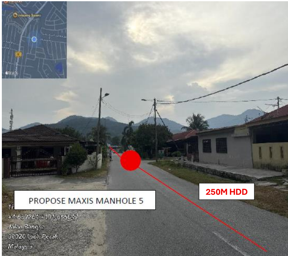
PICTURE 3 : PROPOSE 250M HDD TO PROP MH05
