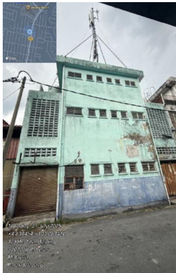
PICTURE 8 : EXISTING MH BUILDING
