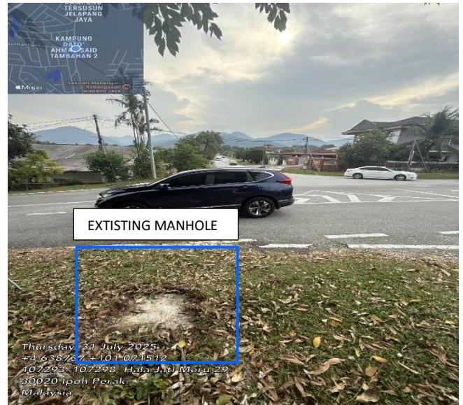
Picture 6 – EXISTING MAXIS M/H
