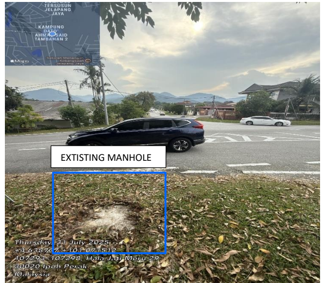
Picture 6 – EXISTING MAXIS M/H
