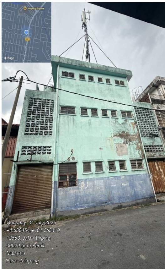
PICTURE 1 - ROOFTOP UMOBILE
