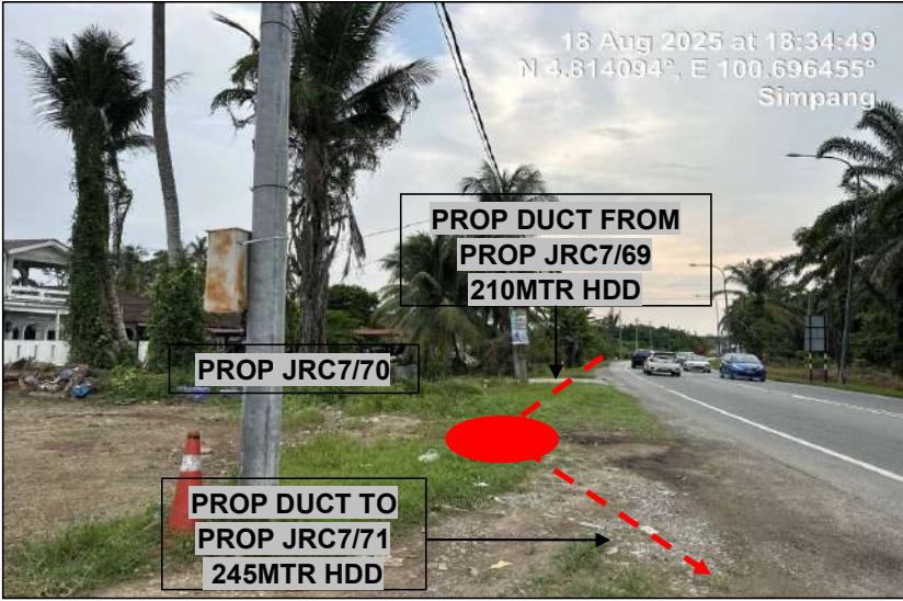
LOCATION AT JALAN TAIPING-KUALA SEPETANG (74)
