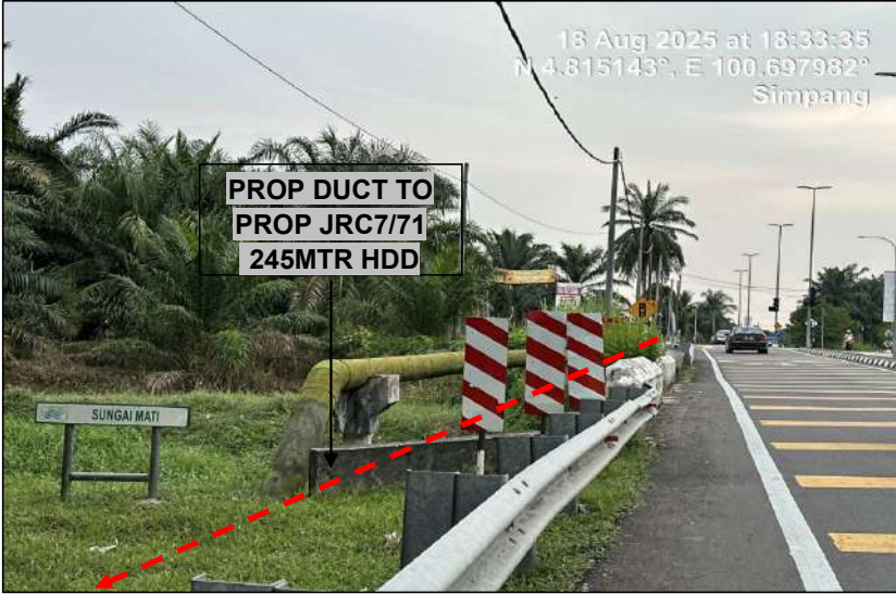
LOCATION AT JALAN TAIPING-KUALA SEPETANG (74)
